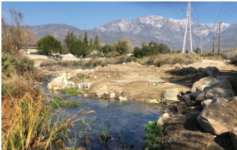
Frankish Tunnel Outfall
