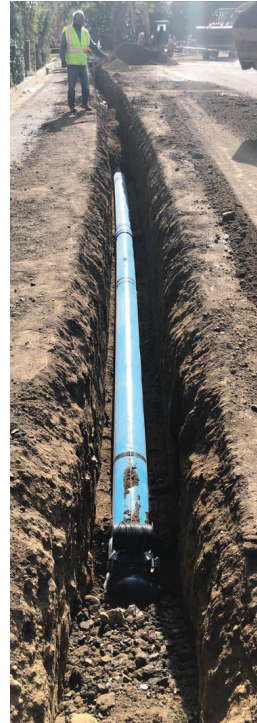
Euclid Crescent Pipeline
